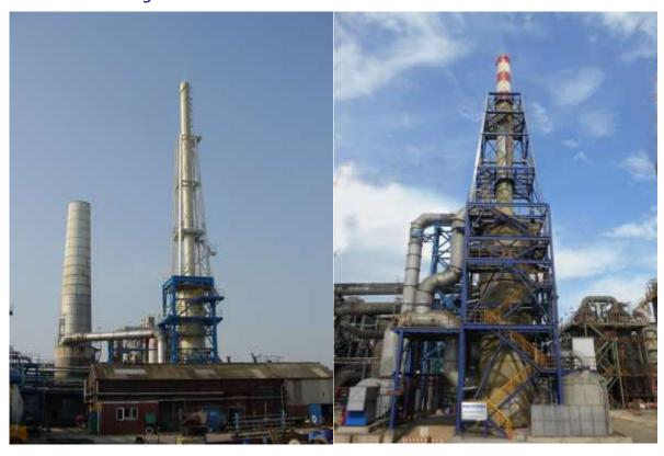
Pic. 18: SUPER<sup>OX</sup>-Processes downstream sulphuric acid plants
