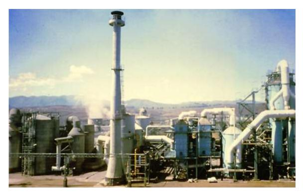
Pic. 11: Cu-smelting based metallurgical DC-plant original 900 tpd and lately revamped to 1,500 tpd
