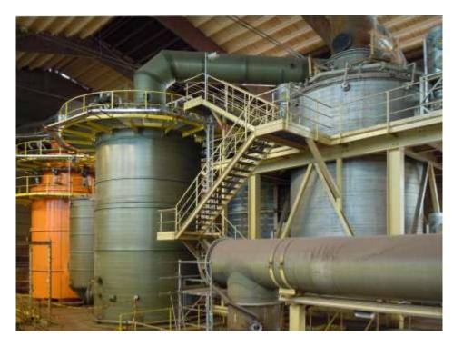
Pic. 6: Complex multistage wet scrubbing unit installed at a metallurgical plant.
