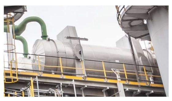
Pic. 16: Anodic-Protected-Acid-Coolers
