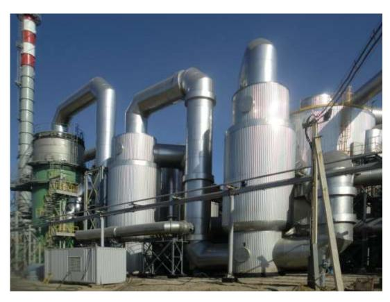
Pic. 7: 2,000 tpd Sulphuric Acid DC-Plant based on sulphur burning with THRC
